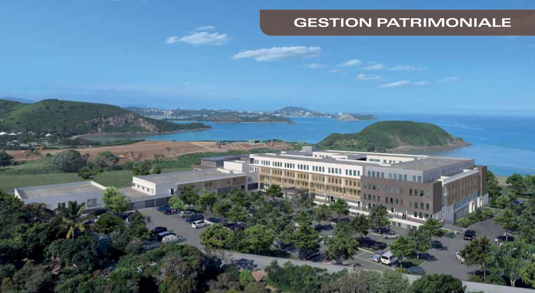
Clinique de Nouville - Nouméa - SANAE Architecture - Artelia
